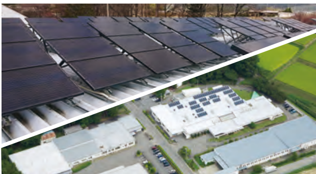
Installation of solar power panels (Logitec INA Solutions, Ina Factory)
