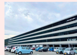
Hyogo Logistics Center, ELECOM
